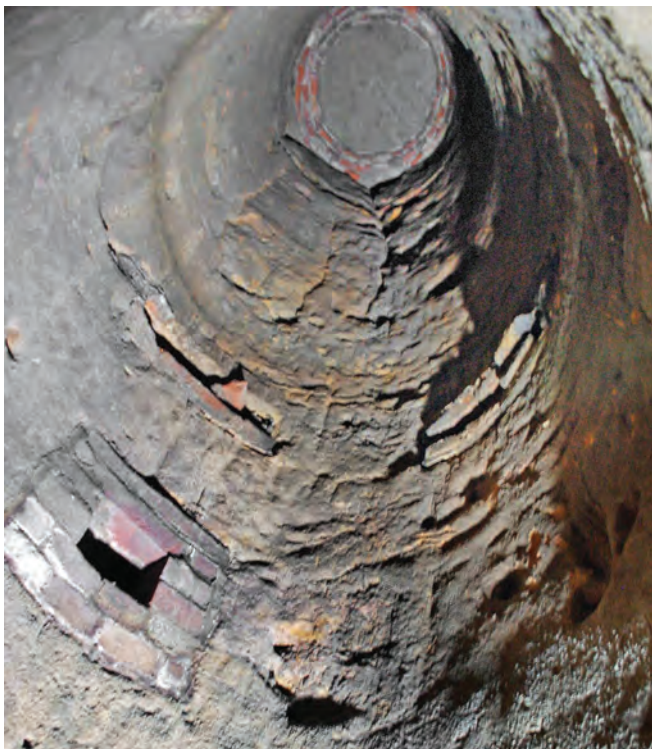
Looking up the well
